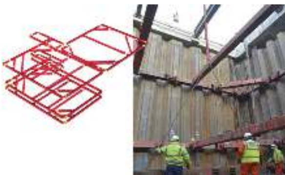
Figure 4. Image of cofferdam installation in progress with BIM model of frame [15]
